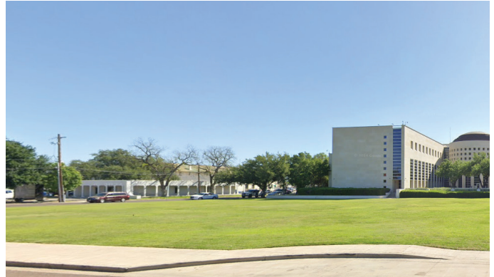
Figure 4. George P. Kazen Federal Building
