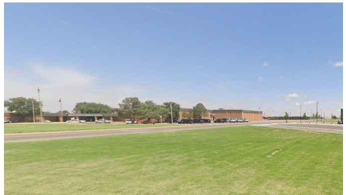
Figure 5. Brownfield Middle and High School
